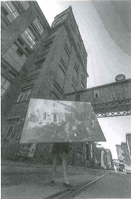
The "Alte Spinnerei" in Leipzig is a huge complex of artist studios and galleries in a complex of old industrial buildings that once housed the largest cotton mill factory in continental Europe. (Saxony Tourism/LTM-Peter Hirth)
